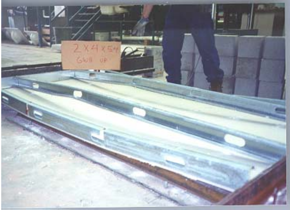
FIGURE 5 Failure of a 2x4x54 mil wall stud due to local buckling of the compression flange at a web punch-out with a 25 psf or 50 psf lateral load (sheathing has been removed).
