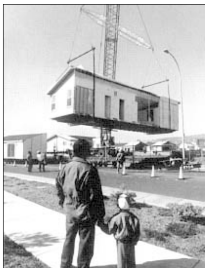
Figure 2.1: Manufactured housing is transferred to the construction site and lowered onto its foundation Source: HUD
