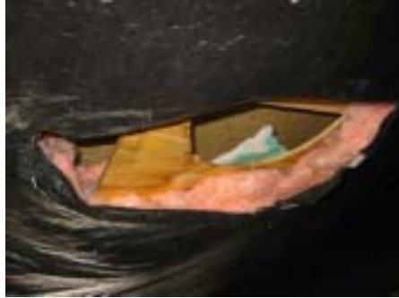
Figure 2-12 Bottom board hole in single section home
