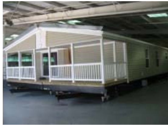
Figure 2-2 Double section test home
