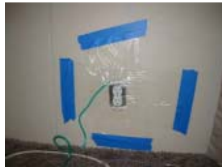
Figure 2-6 Pressure probe in wall
