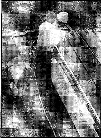
Fig. 2. PV roof modules being installed.
