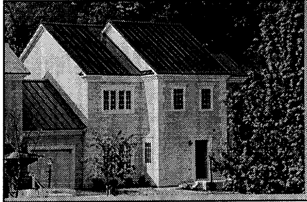
Photovoltaic roof on a Twenty-First Century Townhouse in the NAHB Research Home Park, Bowie, Maryland
