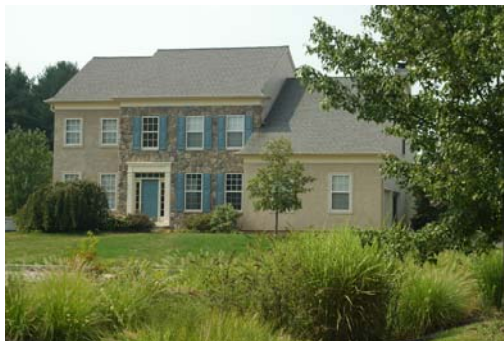
Figure 3. Field Investigation. Single-family Residence in Ambler, PA
