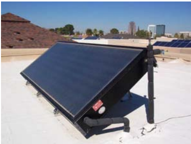
Reflective Roof Coating
