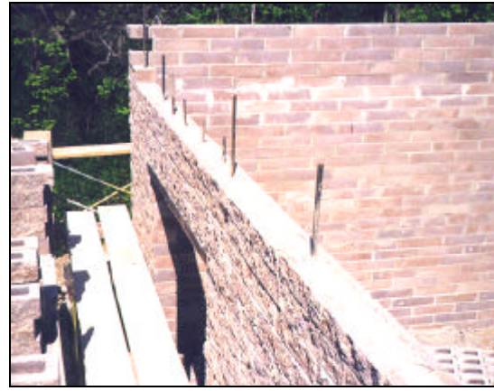
Photo 4. Bond Beam at Minnesota Site
