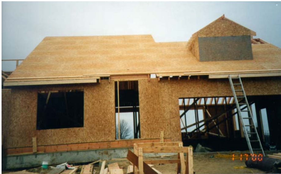
Wood House Framing
