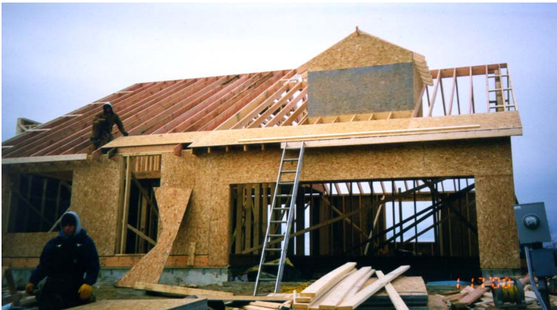
Wood House Wall Framing
