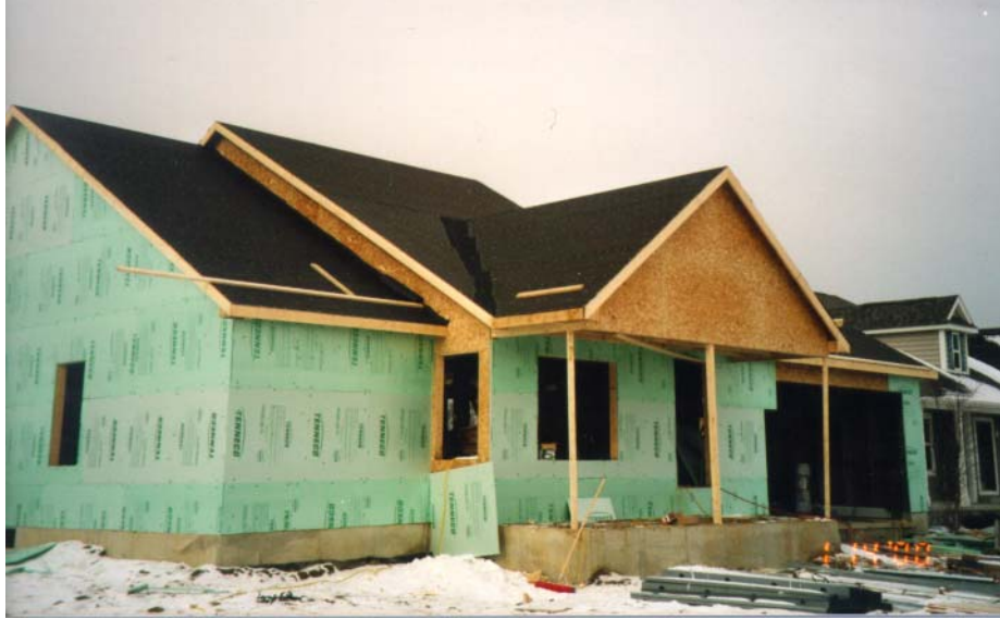
Steel House Framing
