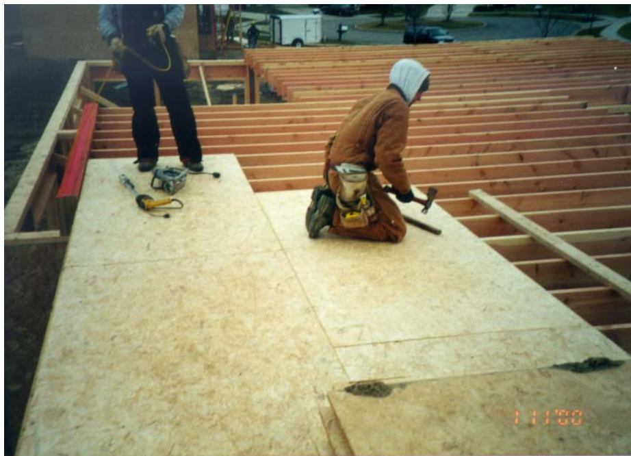
Wood House Floor Framing
