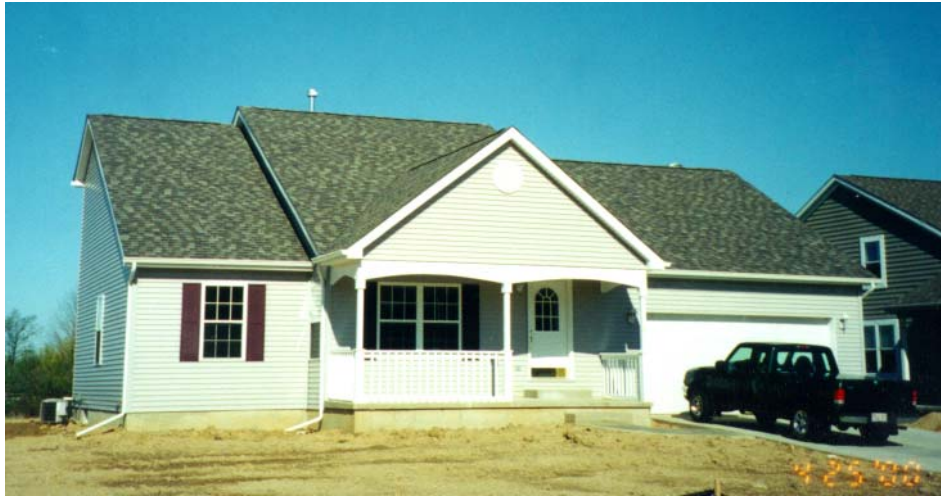
Finished Steel House
