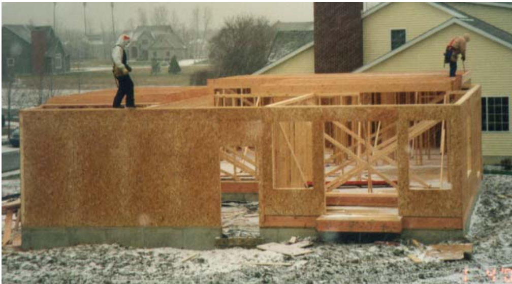
Wood House Wall Framing
