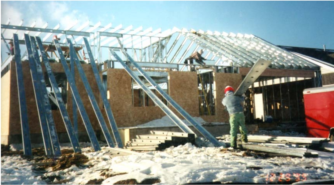
Steel House Roof Framing
