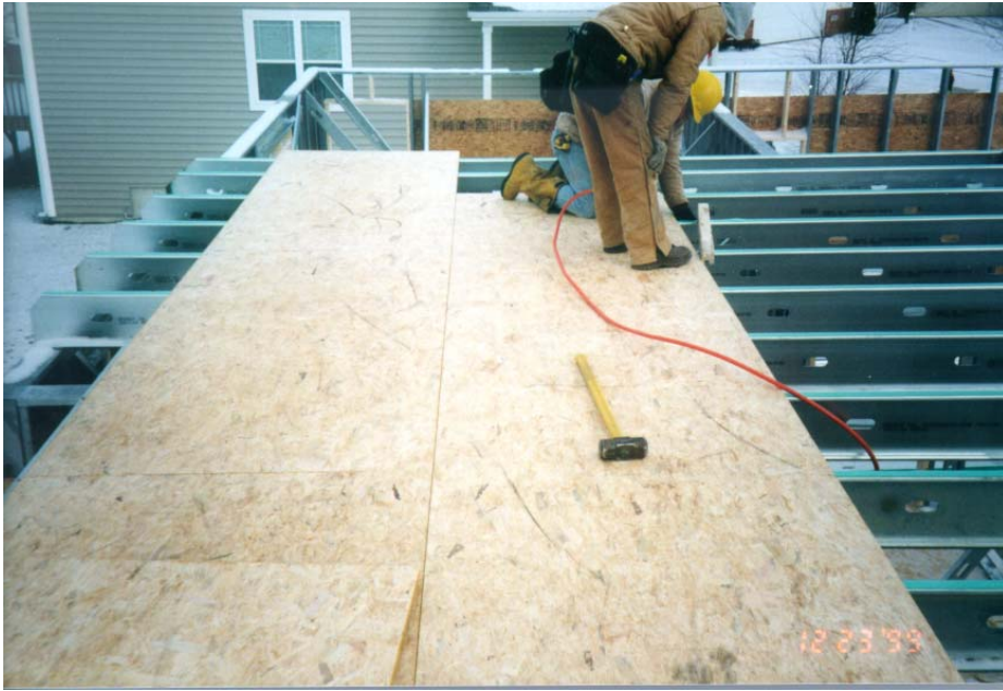
Steel House Floor Framing
