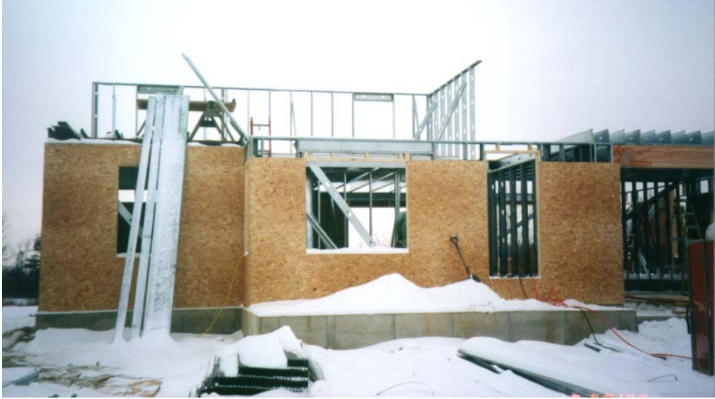
Steel House Wall Framing
