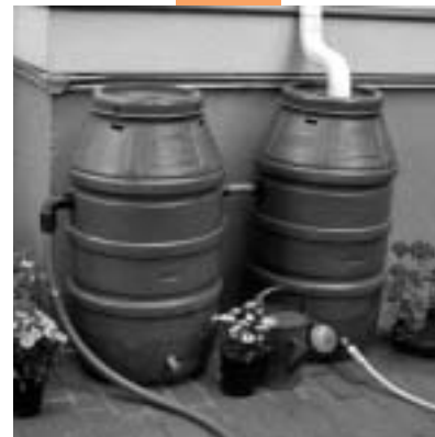
Fig. 4-43a and Fig. 4-43b Rain barrels used to capture rainwater from roofs. Rain barrels can be connected to provide more storage capacity.
