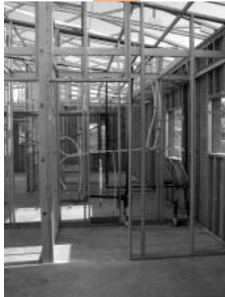
Fig. 4-16b Interior steel framing, Primavera Builders, Tucson, AZ.
