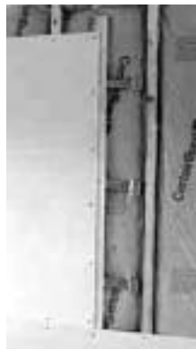
Fig. 4-41a Drywall butt joint system.
