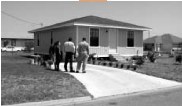
Fig. 4-1 Sidewalks were eliminated in this project by non-profit developer Proyecto Azteca, San Juan, Texas
