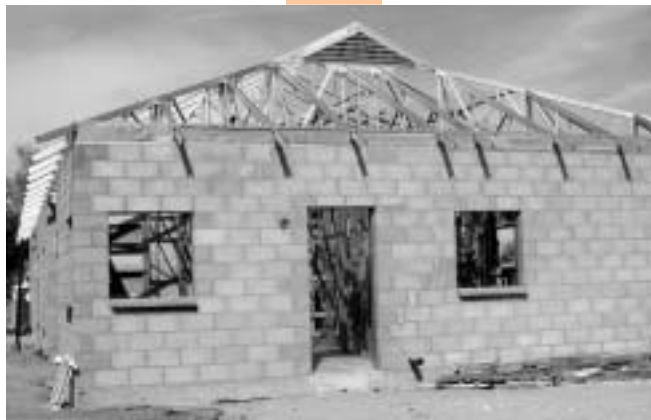
Fig. 4-16a Steel-framed metal roof, Primavera Builders, Tucson, AZ
