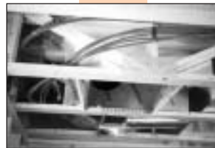
Fig. 4-33 Open-web floor joists make the installation easier.
