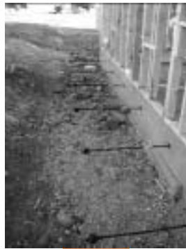
Fig. 4-10 Post-tension slabs-on-grade were used for homes in a rural subdivision with poor soil in Arizona. Life Rebuilders, Superior, AZ
