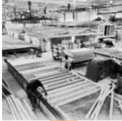
Fig. 4-6 Manufactured homes are constructed in factory-controlled conditions
