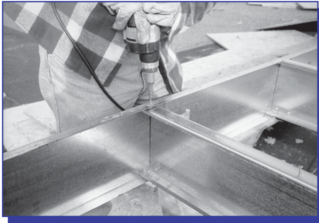
Figure 6.3. Fastening Track to Joist
