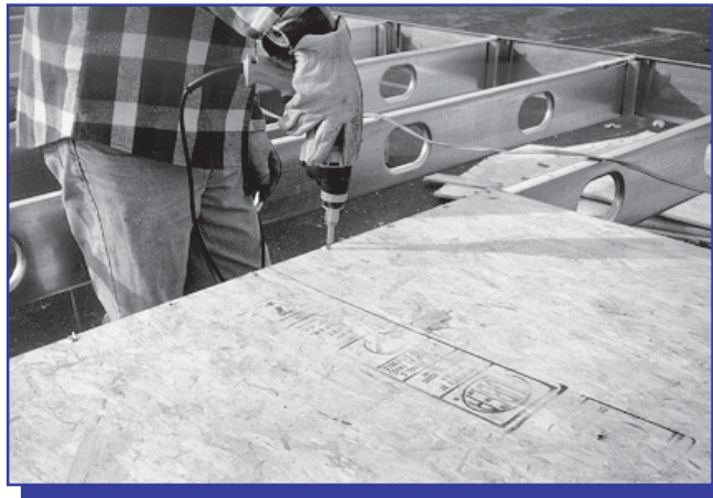
Figure 6.4. Fastening Panel Ends
