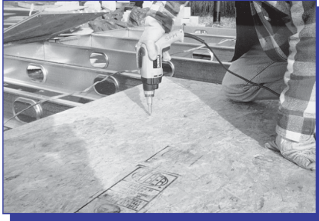
Figure 6.5. Fastening Sheathing to Steel Joists
