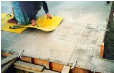
Concrete stamping, K. Hovnanian Field Evaluation
