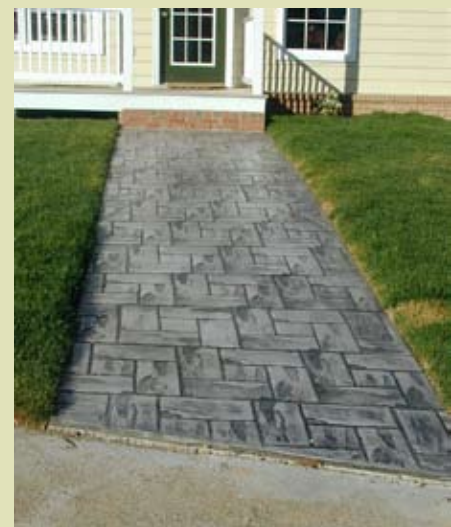
Stamped concrete walkway, MADE Homes Field Evaluation
