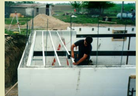
Hopke Buildings and Grounds Field Evaluation
