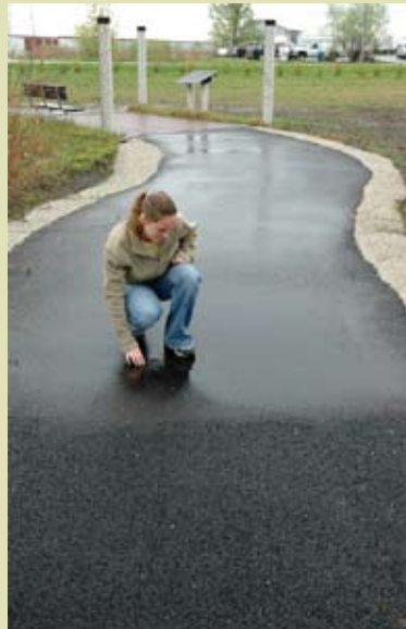
Above left: Difference between permeable asphalt and impermeable asphalt laid side by side for comparison. Above right: Permeable asphalt allows water to seep through.
