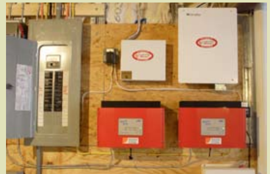
PV Inverter and electric panel interface, Source: 2007 EVHA Silver Award Winner Bob Ward Companies
