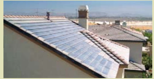
Roof integrated PV panels, Source: 2005 EVHA Gold Award Winner Pardee Homes
