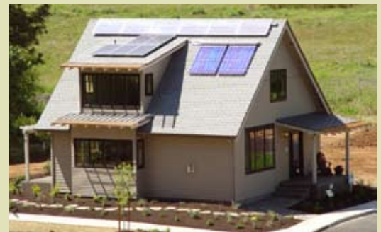
Roof mounted PV system along with solar hot water heating coil (lower right panels), Source: 2008 EVHA Silver Award Winner Sustainable Development, Inc.
