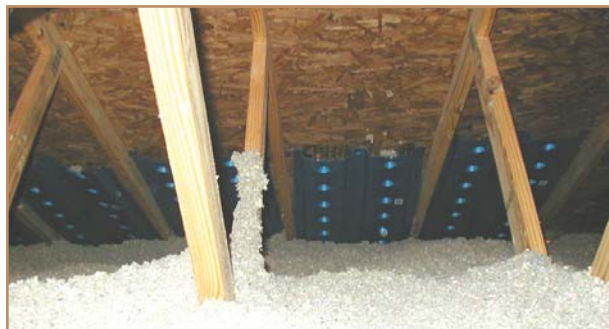
Adding attic insulation while maintaining proper ventilation can improve comfort, lower energy bills, and reduce moisture-related roofing problems.
