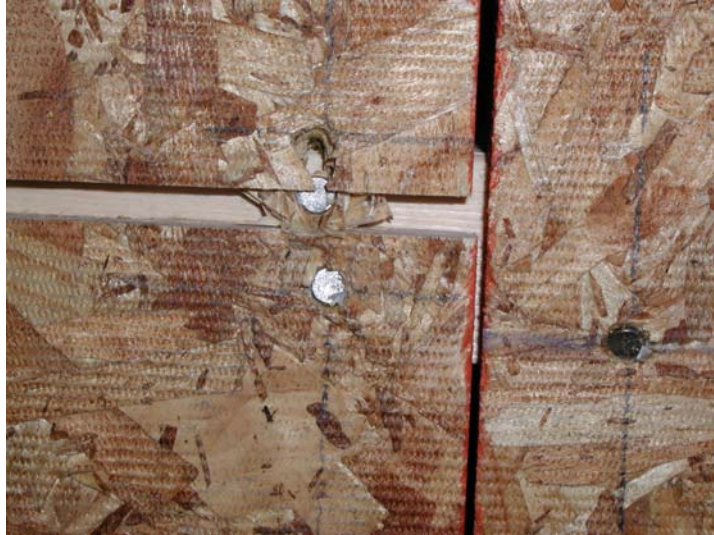
Figure 3.7 – Fastener tear-through failure at region E
