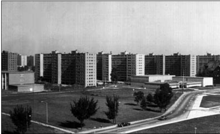
Figure I-1: Overall view of Pruitt-Igoe, a 2,740-unit public housing project constructed in St. Louis in the 1960s.
