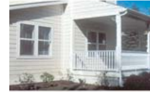
Site-built porches lend scale to factory-built homes (courtesy, MHI).
