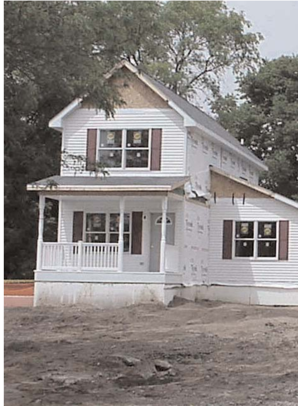
Modular units feature site-built porches and steep-pitch roofs (courtesy, Rural Housing Institute).
