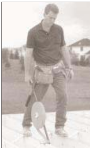
INSTALLING FOAM GASKET
