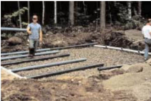
DRAINFIELD INSTALLATION
