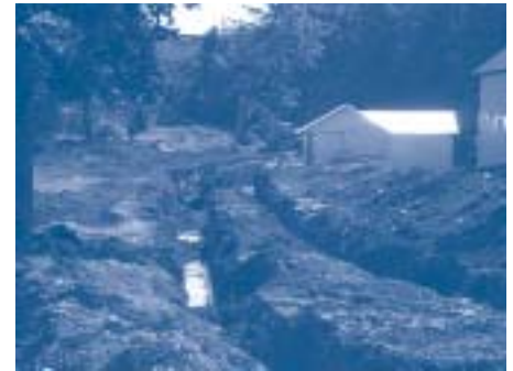
Horizontal trench for geothermal loop to heat exchange with the ground
