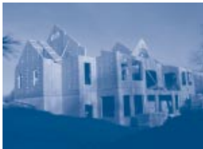
Engineered panels, such as SIPs, can help reduce energy and labor costs, but may cost more up front.
