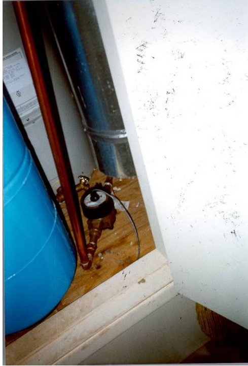
Figure A5 Inside the house, the research water meter monitors whole house water use.
