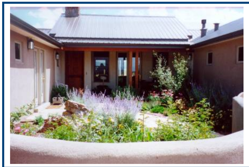
Figure 12 Front courtyard irrigated from rainwater system
