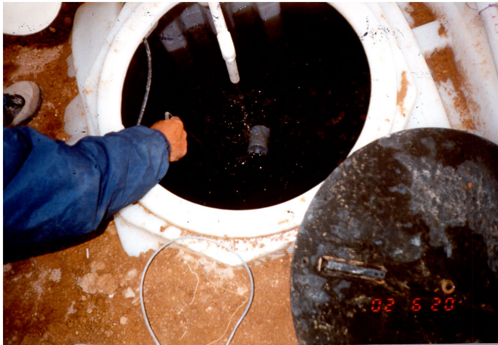
Figure A4 Adjusting the float switch in the new rainwater tank.
