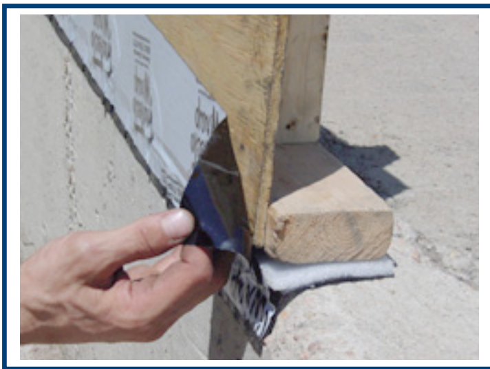
Figure 3 - Protecto Wrap® sill plate seal with integral adhesive for an air and water seal
