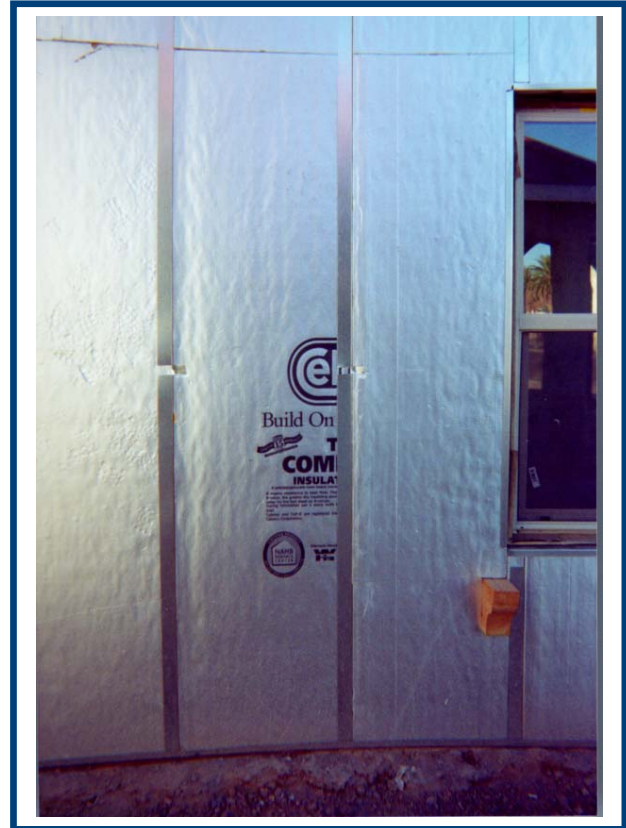
Figure 5: Example of wall insulation
