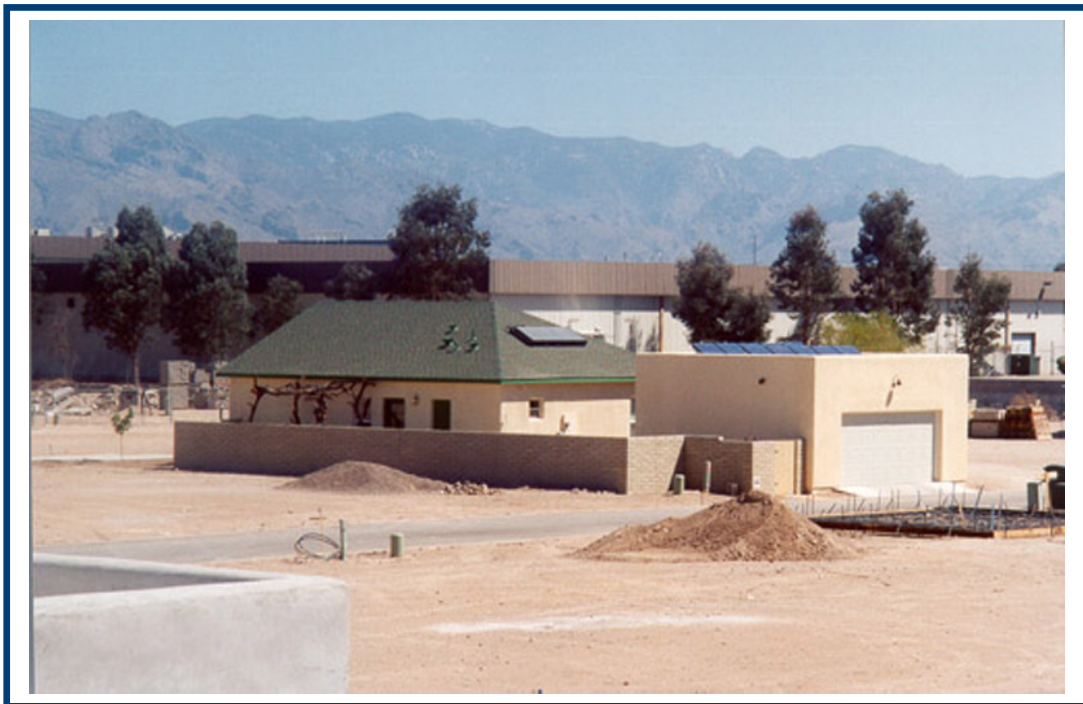
Figure 6: House A with solar PV and hot water systems
