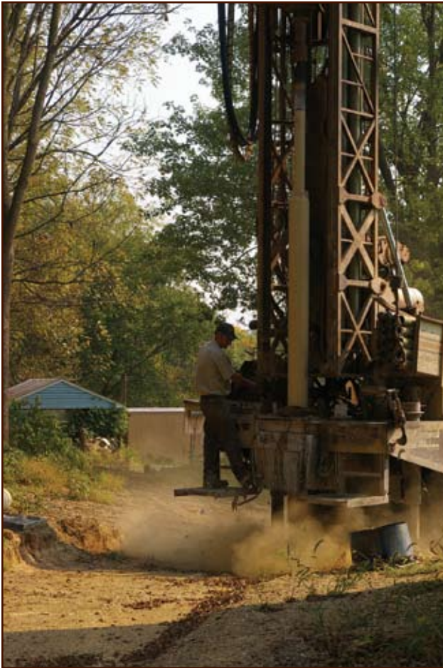
A geothermal system provides high-efficiency heating and cooling.
