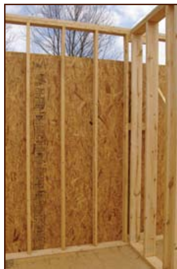
OVE framing techniques improve the insulating value of exterior walls.
