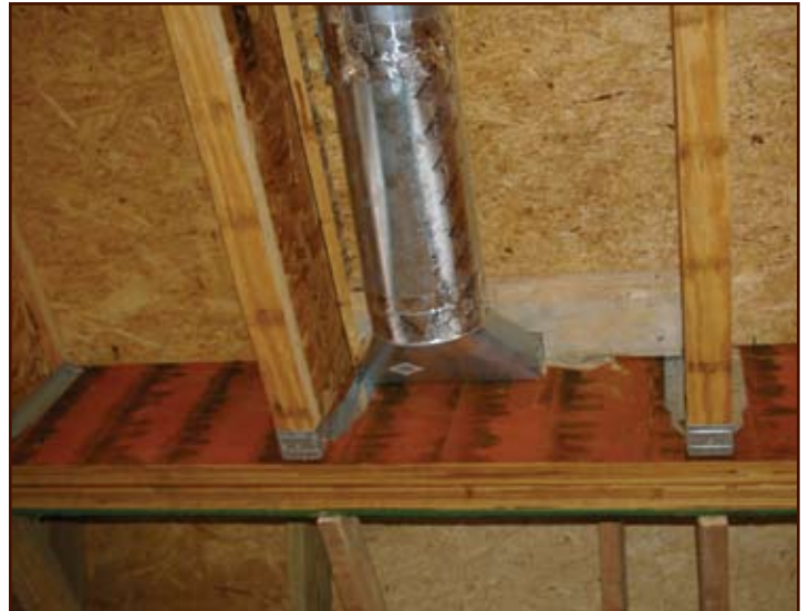
Foil mastic, which is backed with butyl rubber, provides an excellent seal while being relatively simple to install.
