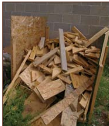
Nearby marked bins facilitate the sorting of recyclable construction waste.
